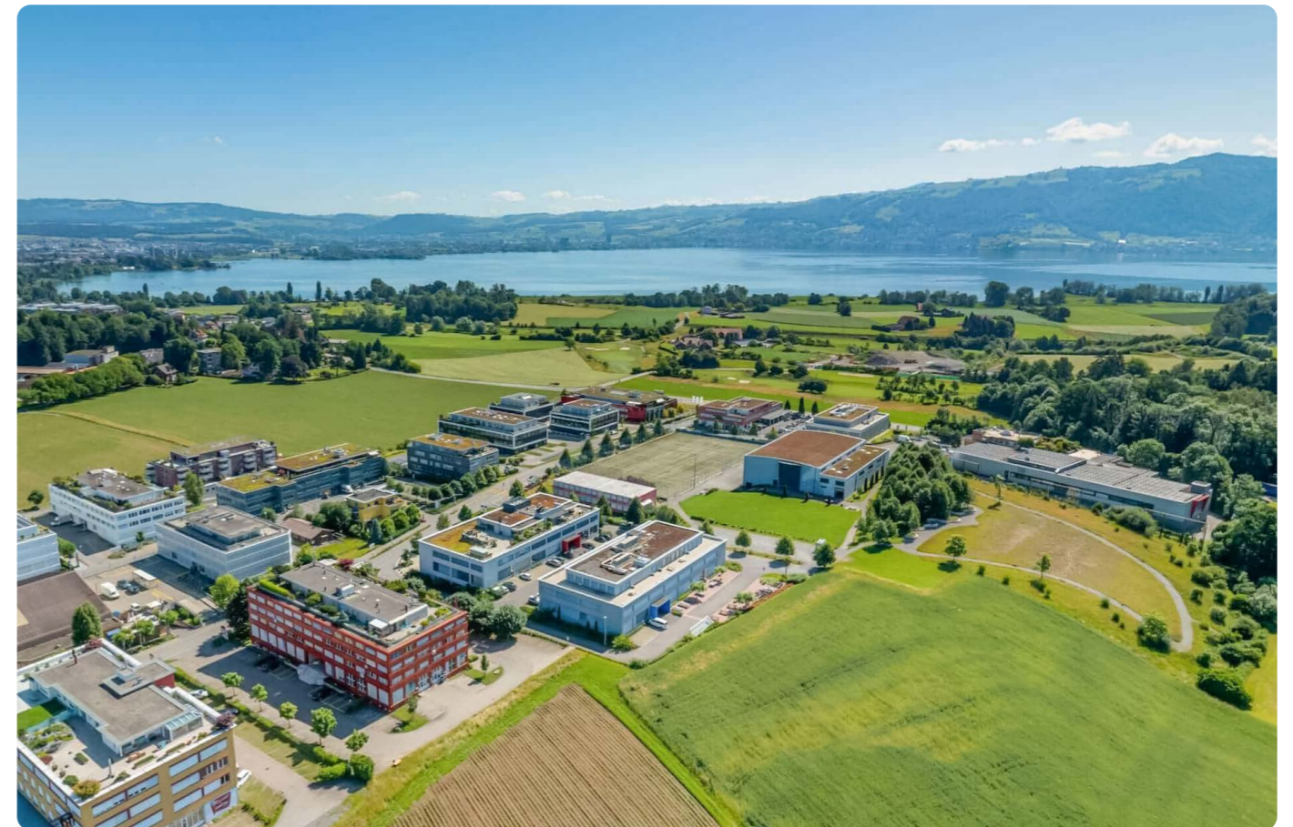
International School in Hünenberg
